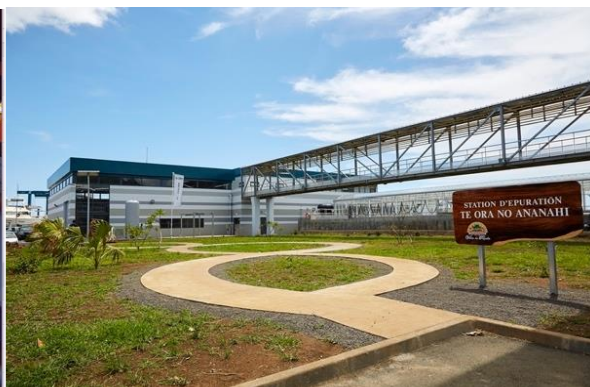
Station d'épuration Te Ora no Ananahi à Fare Ute
